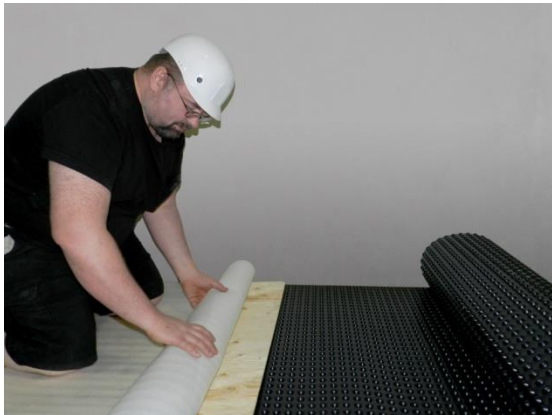
Lay laminate foam underlayment on top of plywood or OSB.
