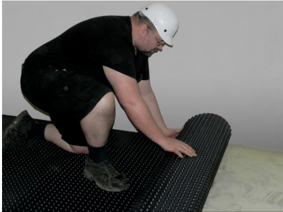
Unroll DMX AG Underlayment™ (dimples facing down).
